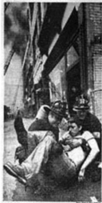
The scene after the fire at the bathhouse in Washington, D.C.
